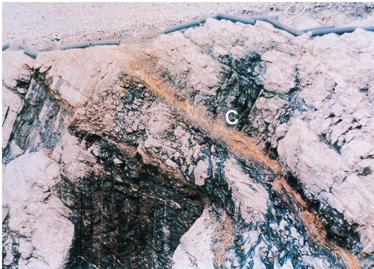
Plate 1. View of northeast and southeast walls of the intake structure showing the 1 m thick yellow-brown southeast dipping shear zone C.
